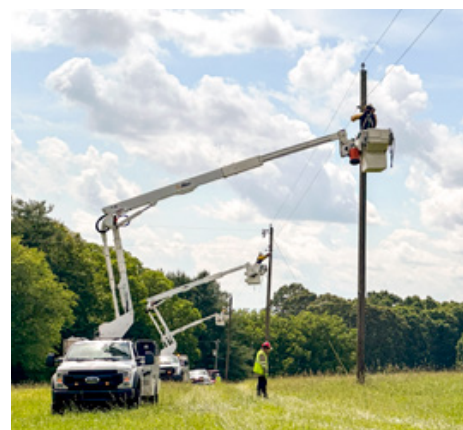
BELOW: Line crews use bucket trucks to pull fiber cables into position.
